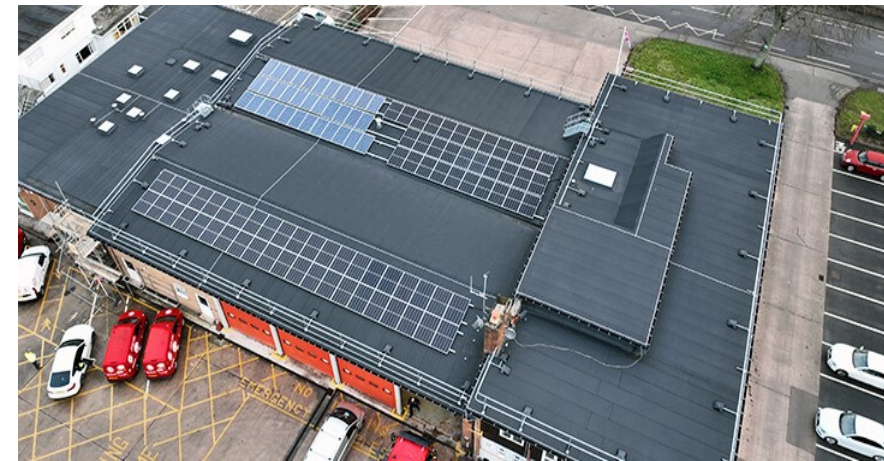
Fig 9 – Example of mineral felt roof with Photovoltaic panels and edge protection
