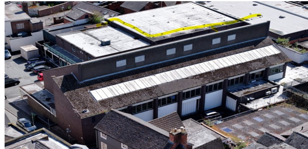
Fig 8 – South and North aerial photos with gas service highlighted
